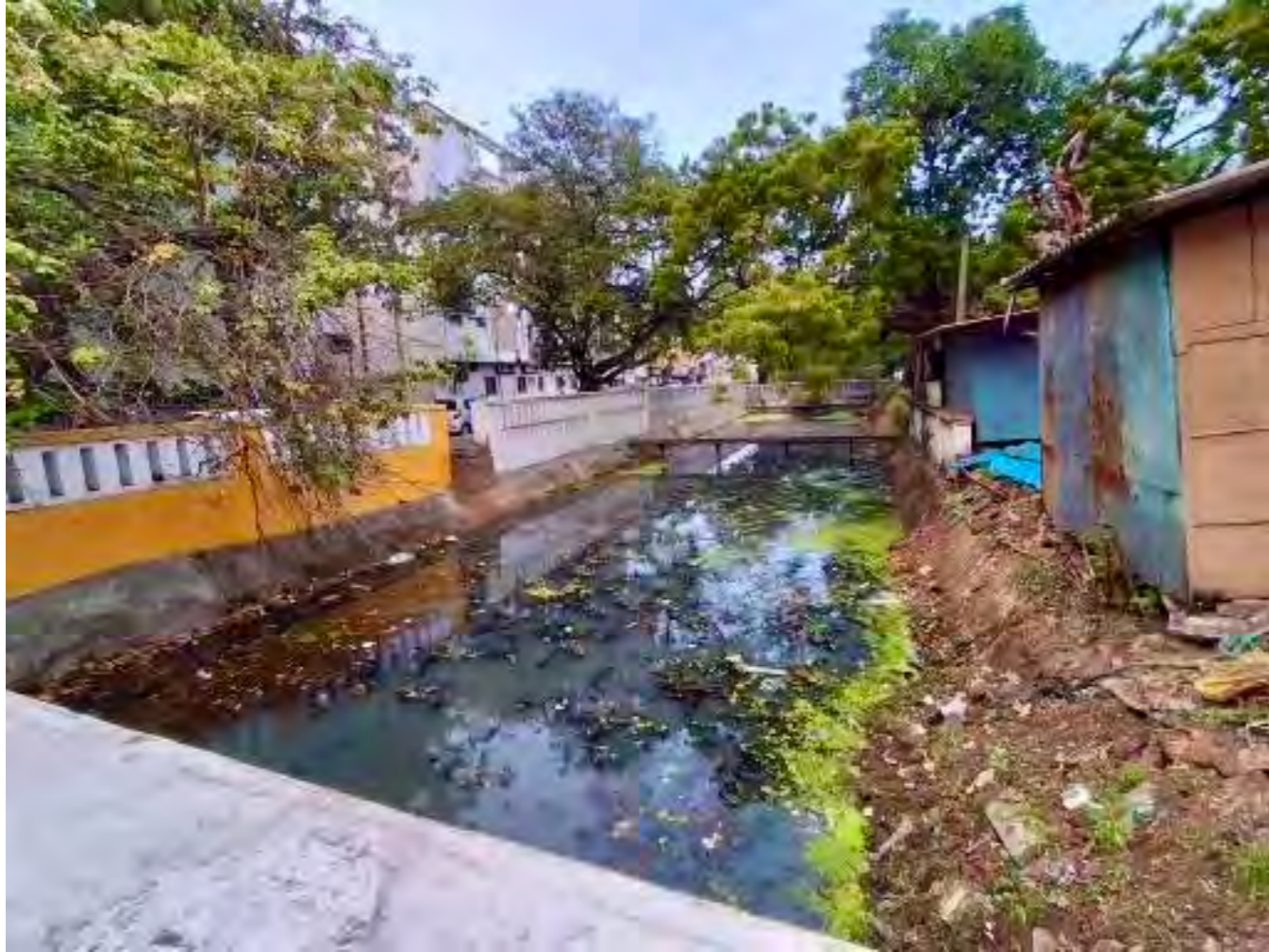
Figure 46. Sewage mixing with the creek and river system
